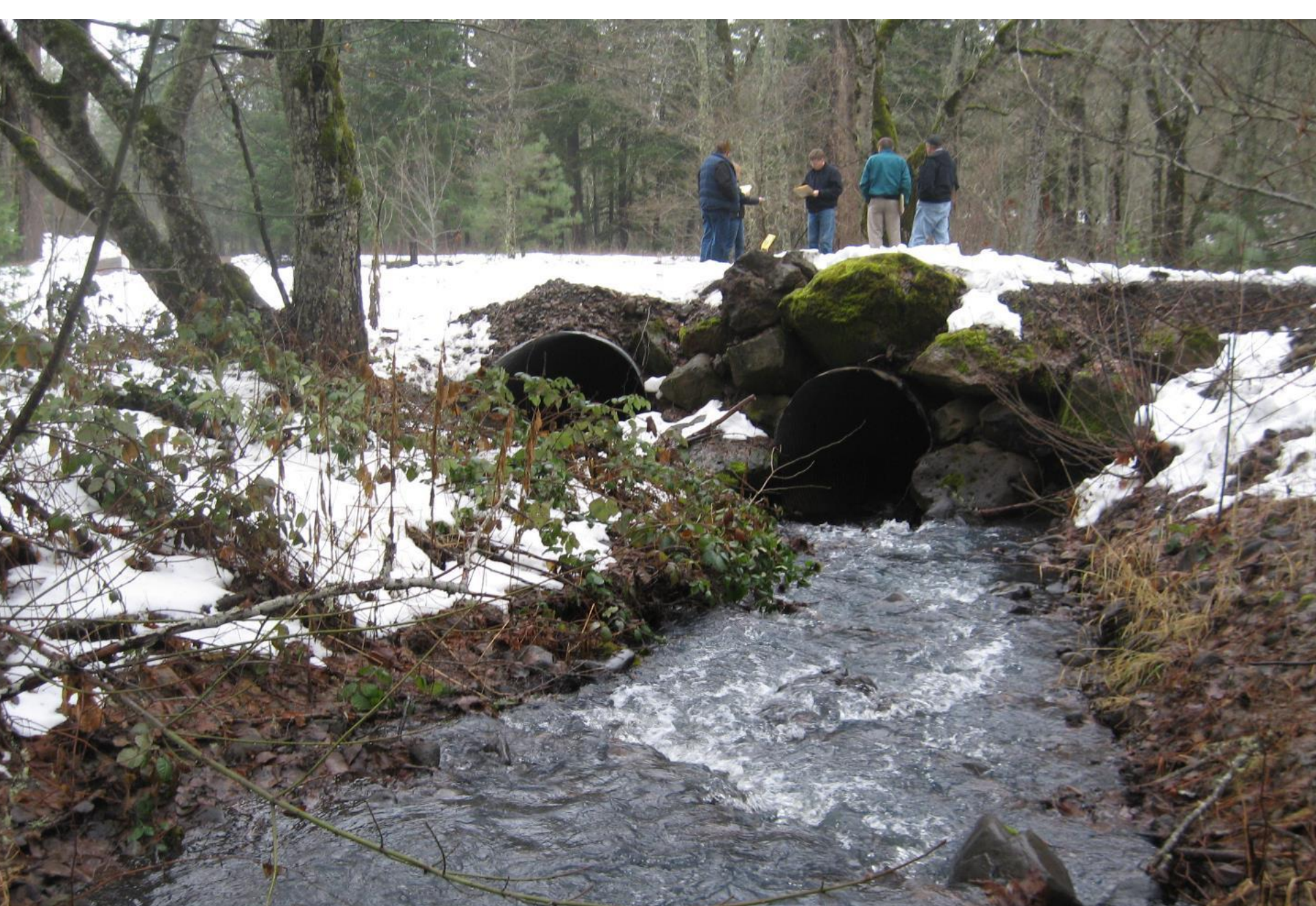
Indian Creek culvert replacement - before
