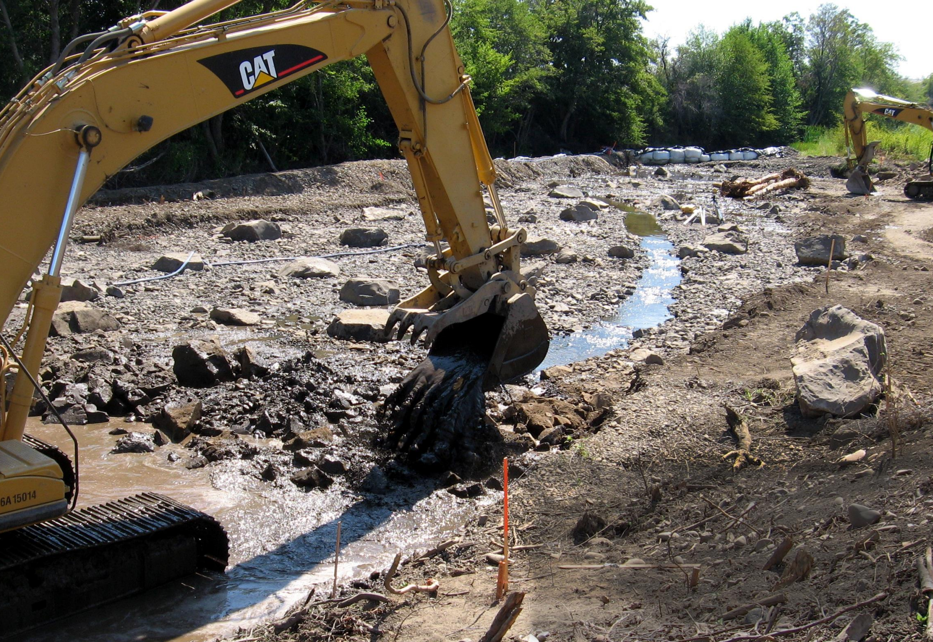
Satus Creek – During Construction
