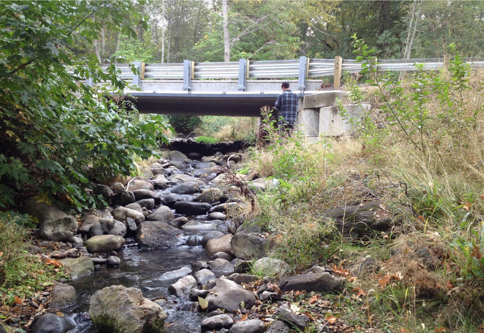
Indian Creek culvert replacement - after
